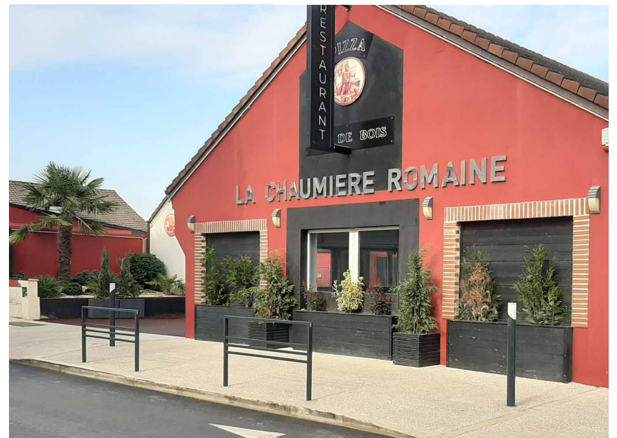
3300 barriers and 5200 steel bollards Menecy - 91 - France
