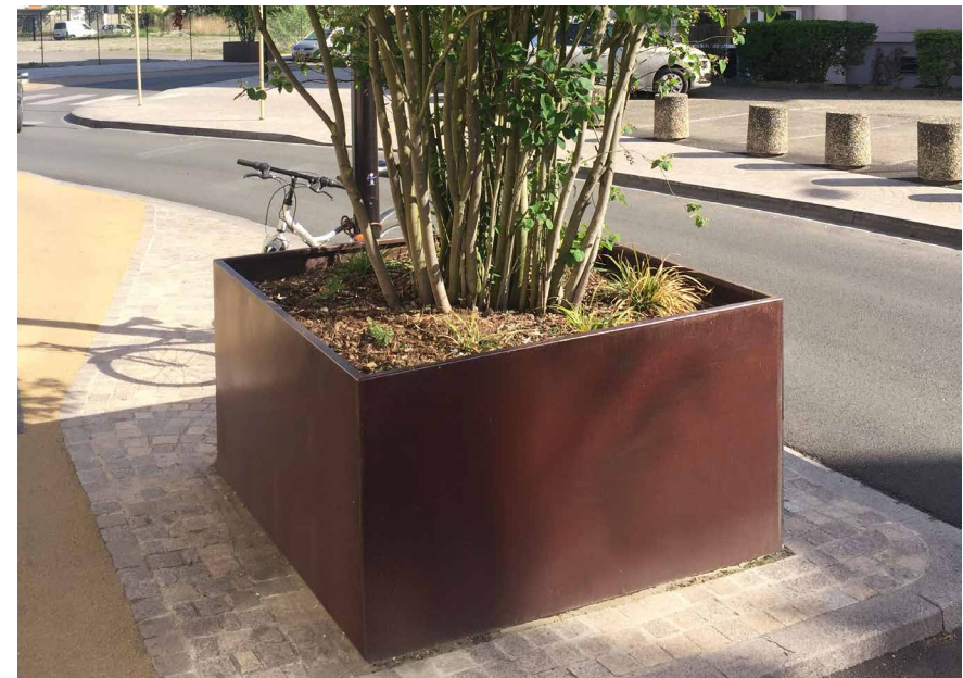
Corten®-type steel earth retainer Colmar - 68 - France
